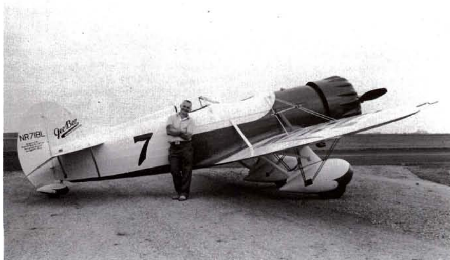
Ken Flaglor strikes a nonchalant pose beside his pride and joy. The Gee Bee is big, with an empty weight of 1,792 lbs. The streamline wires alone weigh 32 lbs.!
